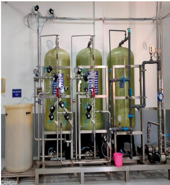
Step 3: Raw water passes through Multi-grade filter Step 4: Further raw water passes through Softener
