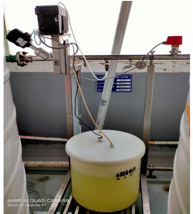
Step 2: NaoCl dosing for Chlorination
