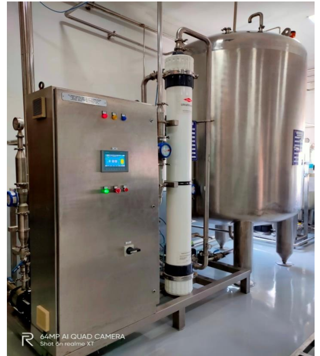
Step 5: Soft water is passed through 150 \mu cartridge filter Step 6: Soft water then passed through Ultra-filtration.
