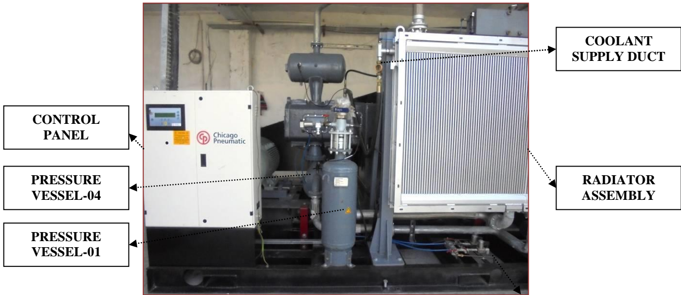
Fig. 02: Key Components of Compressed Air System
