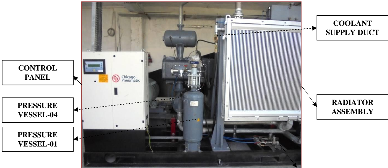
Fig. 02: Key Components of Compressed Air System
