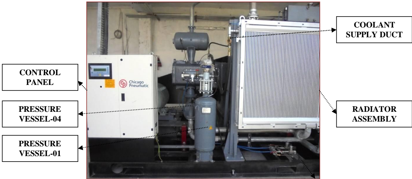
Fig. 02: Key Components of Compressed Air System
