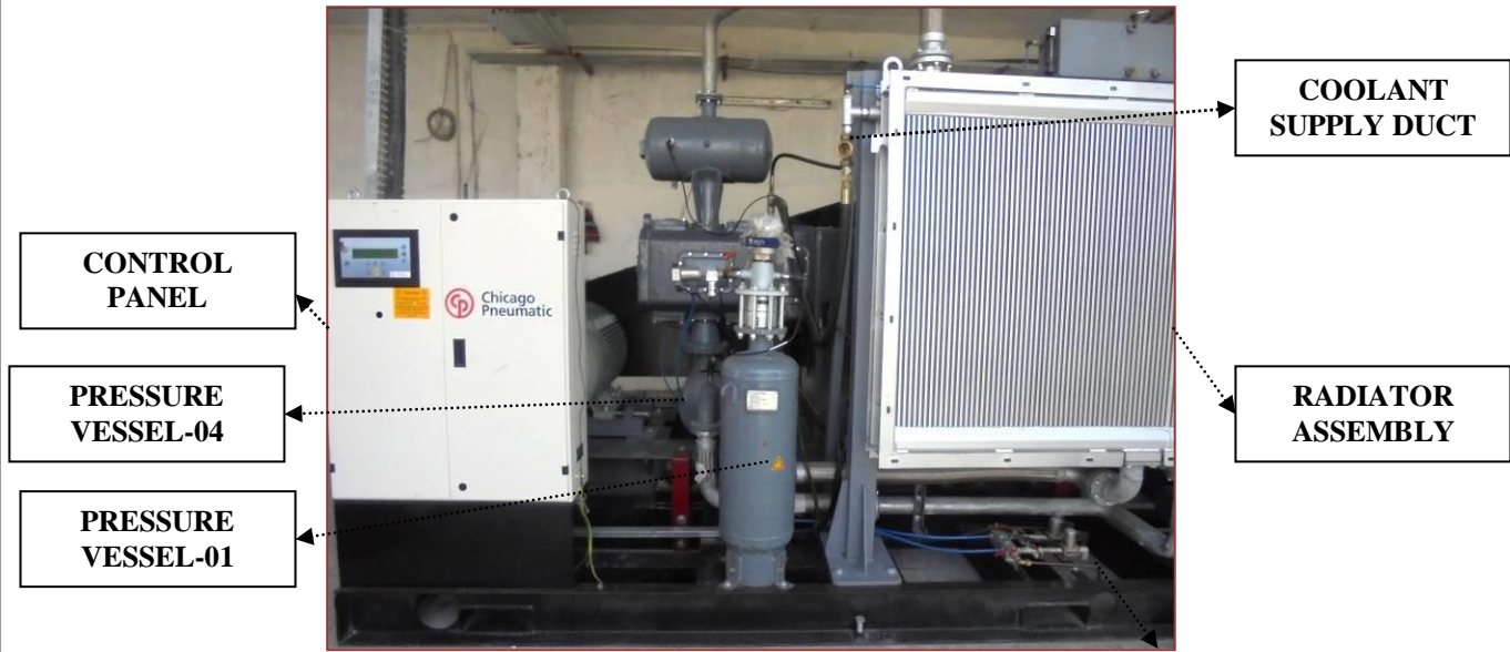
Fig. 02: Key Components of Compressed Air System
