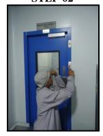
press the door interlocking and enter in air lock-I
