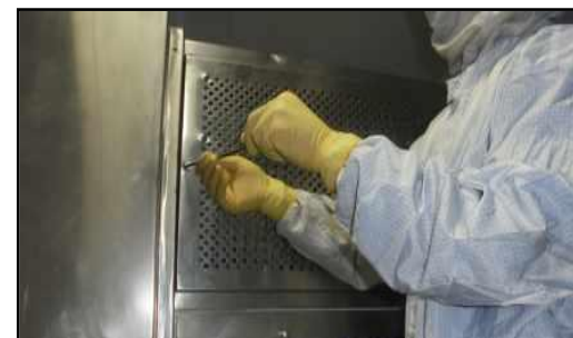
Screw fixing after Pre-filter installation
