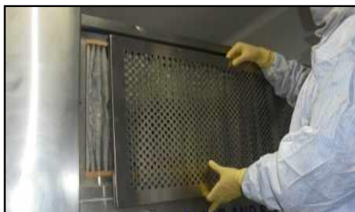
Install Pre-filter grill (after cleaning)
