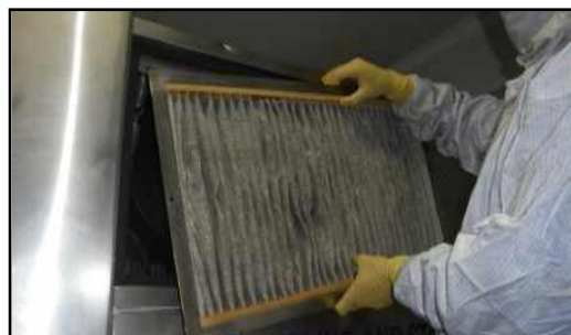
Install Pre-filter (after cleaning)
