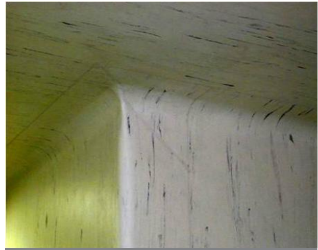
Cleanroom wall and ceiling interfaces with coved and rounded corners
