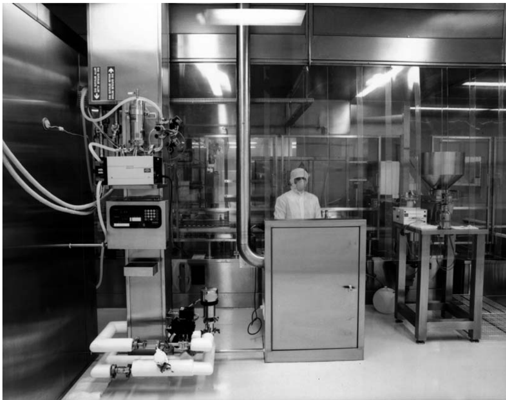
Figure 3.18. Photograph illustrating a typical pharmaceutical clean room and some of the equipment usually therein. Note the presence of a curtain of (transparent) heavy-gauge polyethylene strips (most noticeable directly in front of the operator). These strips box off a grade A laminar flow work station. Product filling into final product containers is undertaken within the grade A zone. The filling process is highly automated, requiring no direct contact between the operator and the product. This minimizes the chances of accidental product contamination by production personnel. Photo courtesy of SmithKline Beecham Biological Services s.a., Belgium
