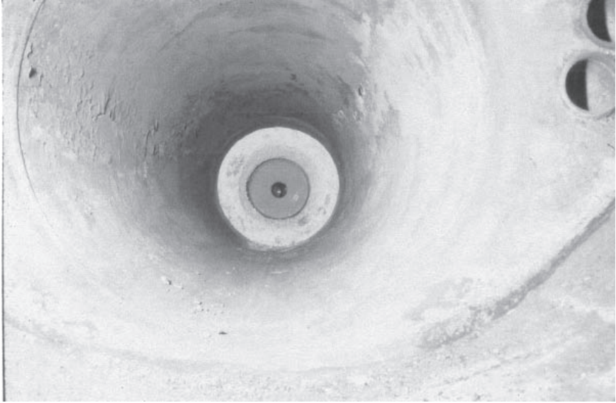
Figure 15-1. Inspecting firing chamber.
