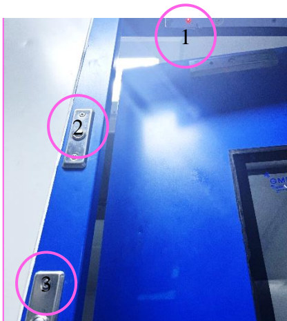
Figure 2: In case of door opening, shows Red indicator Figure 3: Green indicator (Encircled), in case of door closed (Encircled) completely
